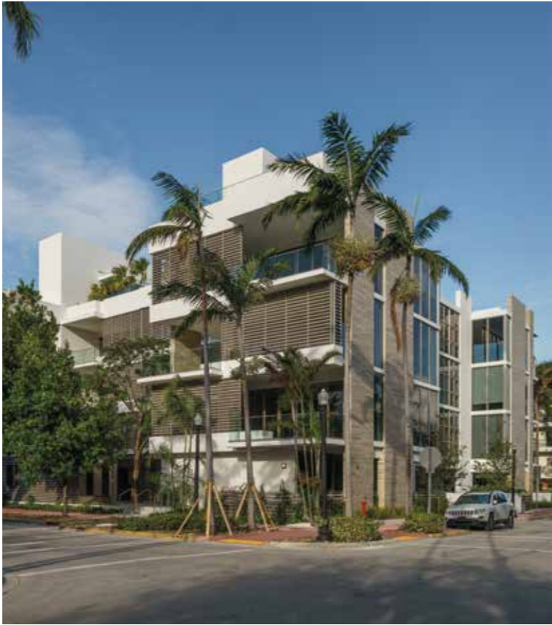
Louver House, Miami, USA
